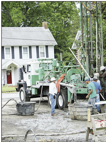
Contractors drilled twenty 300-ft looped wells under the parking lot at St. Philip's, Laurel, for their geothermal heating and air conditioning system. Parishioners, like Len Hickman (foreground) and Fr. Howard Backus (background), put in hours of sweat equity to accomplish the project.
