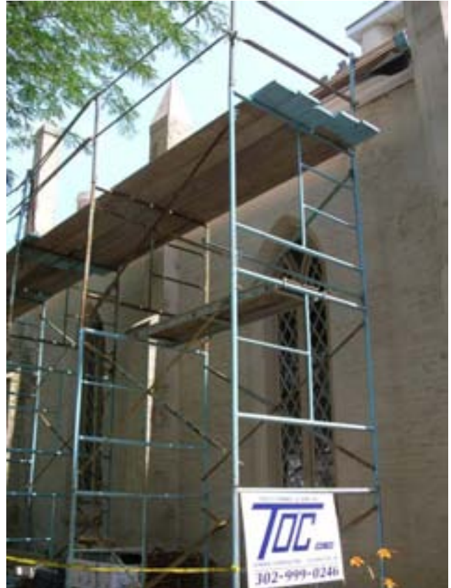
The structural work continues.
